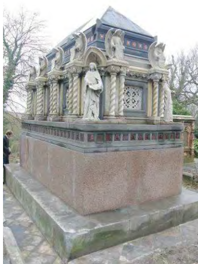
The restored Berens mausoleum
