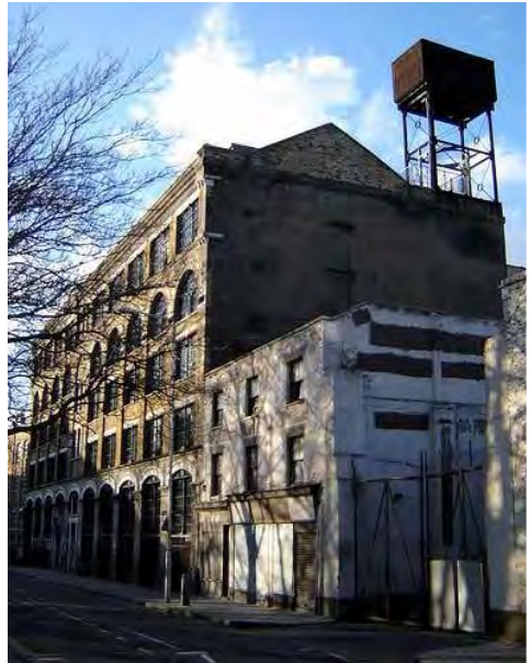
The derelict Barrow, Hepburn & Gale Ltd works in Long Lane, Bermondsey in 2007 7
