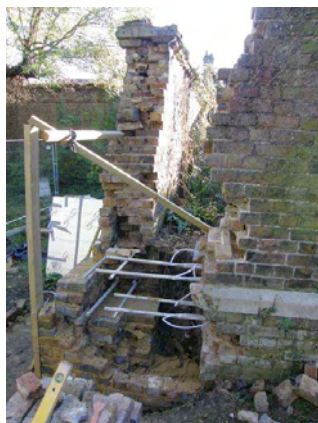
Cemetery wall under repair near to Hubbard Road
