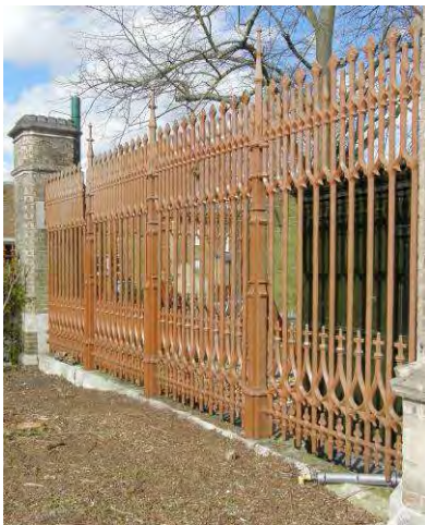
The newly-revealed railings in the Cemetery forecourt
