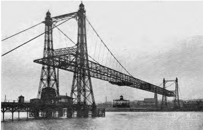
Runcorn–Widnes Transporter Bridge across the Manchester Ship Canal (1905), the first and largest such design
