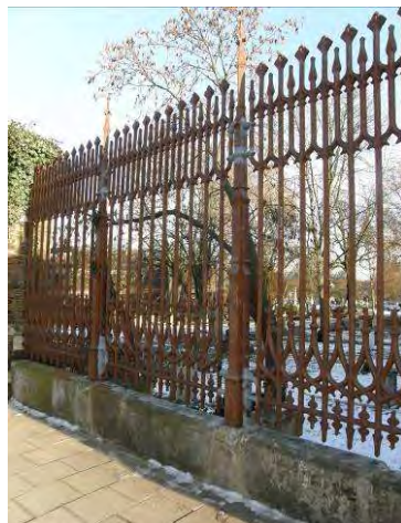
Repaired railings, Norwood High Street
