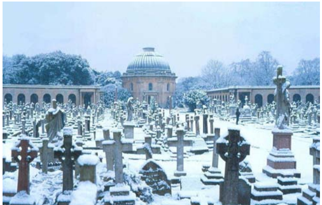
Brompton: General view of the chapel, central area and colonnades (courtesy Robert Stephenson)
