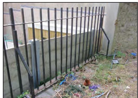
The newly-added wall adjacent to the new housing development (squares 2 & 3)
